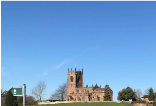
Grade II listed Churchyard wall at Church of St Michael
