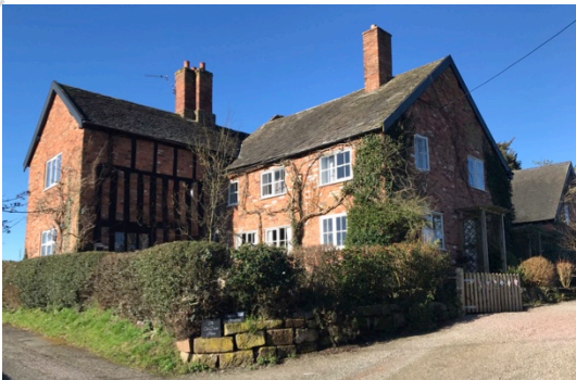
Grade II listed Marbury Cottage
